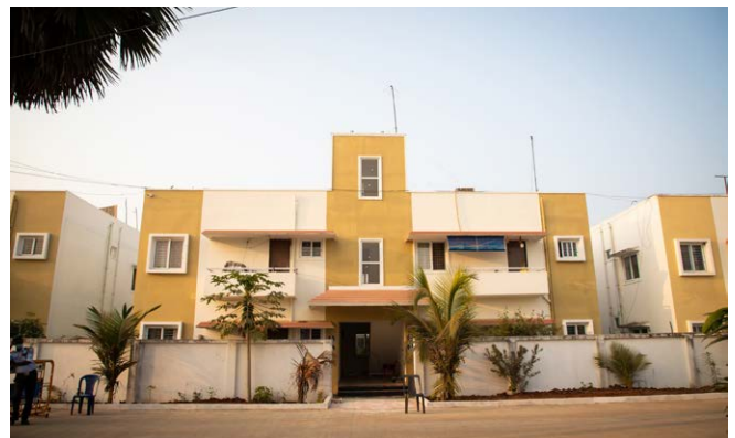
Construction of Rural Housing and Other Rural Development Projects in Antervedipalem, EGDT, A.P.
